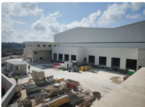
Handaq head office and logistics complex loading bay area March 2026
