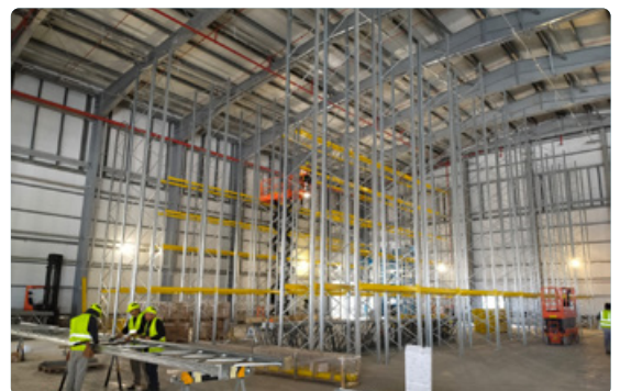
VNA racking system being installed April 2026
